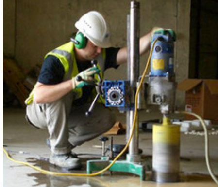
Core sampling to detect chemical contamination in concrete flooring
